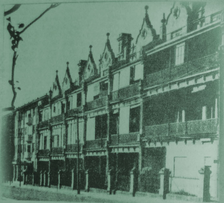
Before the green ban! People's homes, like these in Elizabeth Bay Road, Kings Cross, were demolished and the residents dispersed - to where?
