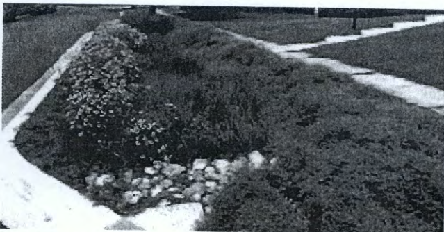
The Amherst Avenue curb extension, completed in December 2014, is a Green Streets project that combined two County interests — keeping local streams healthy and ensuring bus rider safety. The curb was extended into the parking lane and pavement is replaced with plants and soil mix to slow water and filter out pollutants.
