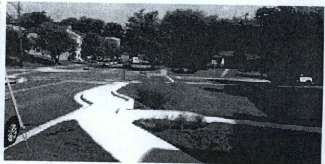
The Amherst Avenue curb extension, completed in December 2014, is a Green Streets project that combined two County interests — keeping local streams healthy and ensuring bus rider safety. The curb was extended into the parking lane and pavement is replaced with plants and soil mix to slow water and filter out pollutants.
