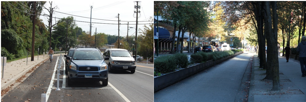
Figure 4: Interim separated bike lanes with flexible delineator posts / parked cars (left) and planters (right)
