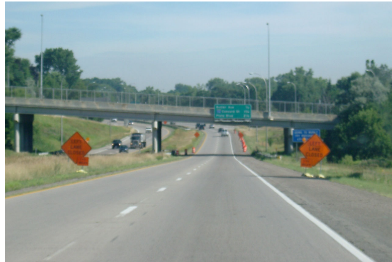
Figure 4.17: US 52 Line of Site Toward the Construction Zone
