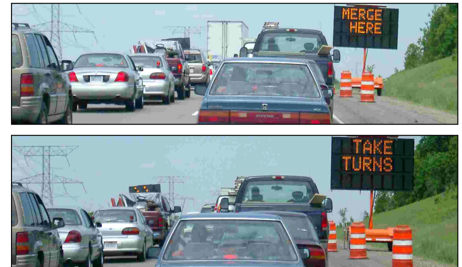
Figure 4.2: Position and Messages Displayed on Last CMS on I-494 NB
