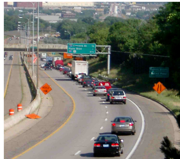
Figure 4.18: US 52 Typical Traffic Pattern During Construction
