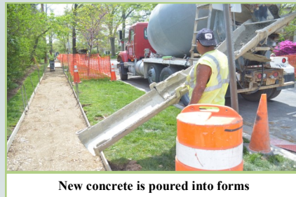
New concrete is poured into forms
