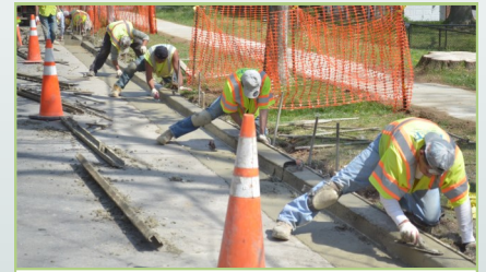
Concrete is smoothed and finished
