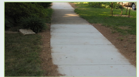
Completed sidewalk repair
