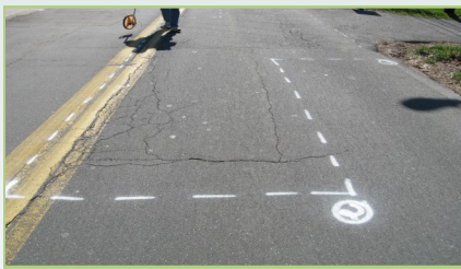
Typical survey paint markings
