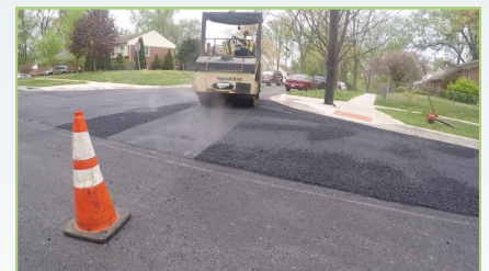
New asphalt is compacted with steel wheeled roller
