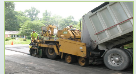
Typical hot mix asphalt paving operation
