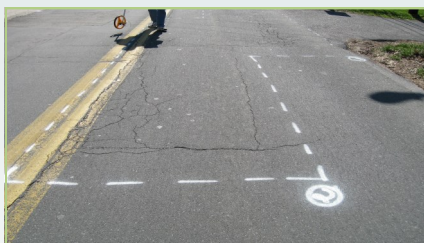
Typical survey paint markings
