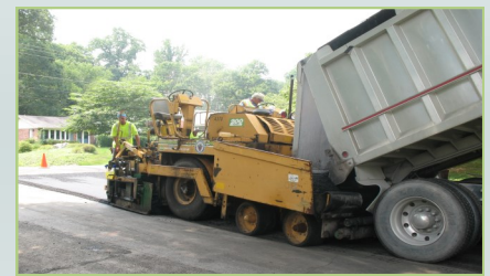
Typical hot mix asphalt paving operation
