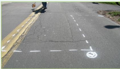
Typical survey paint markings
