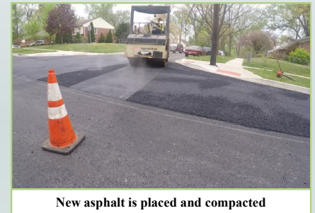
New asphalt is placed and compacted
