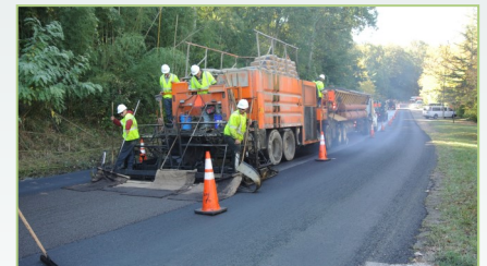
Typical micro-surfacing operation
