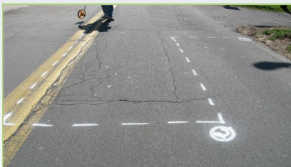
Typical survey paint markings
