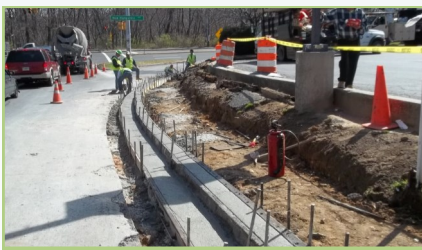
New concrete is poured into forms
