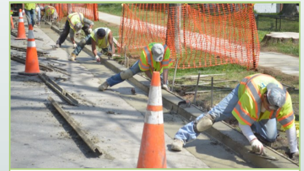
Concrete is smoothed and finished
