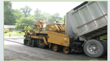
Typical hot mix asphalt paving operation
