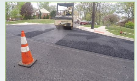
New asphalt is compacted with steel wheeled roller
