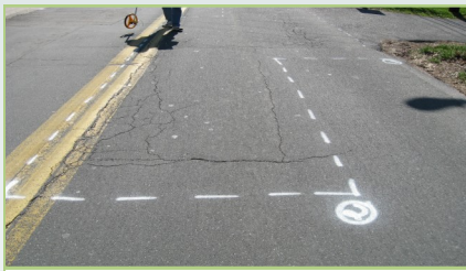
Typical survey paint markings
