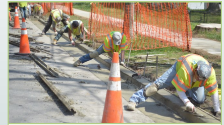
Concrete is smoothed and finished
