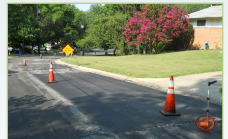
New patch is flush with existing pavement
