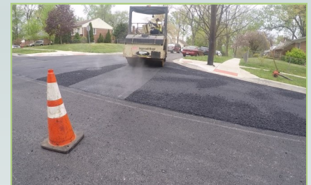
New asphalt is placed and compacted
