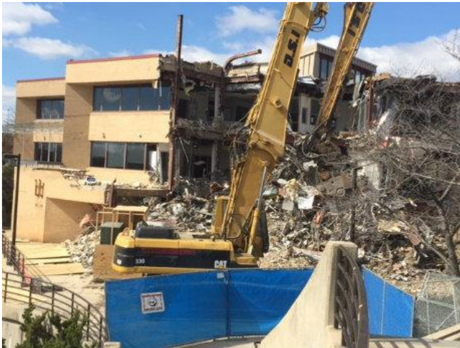
RSC Demolition Progress
