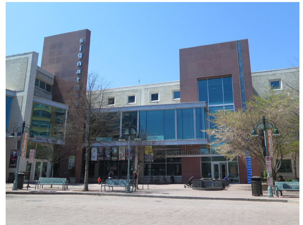
Signature Theater and connected Library
