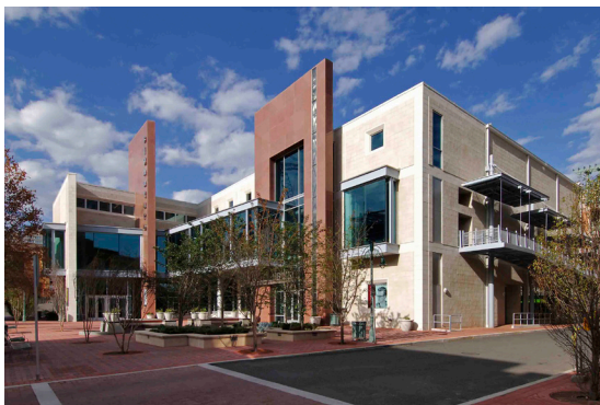
Theater, library and plaza complex
