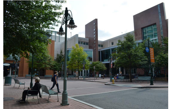
Theater, library and plaza complex
