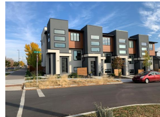
Rowhouses in Killarney along the 37 Street Main Street
