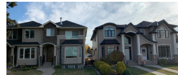
Semi-detached homes, like these in Killarney, would be supported throughout the area
