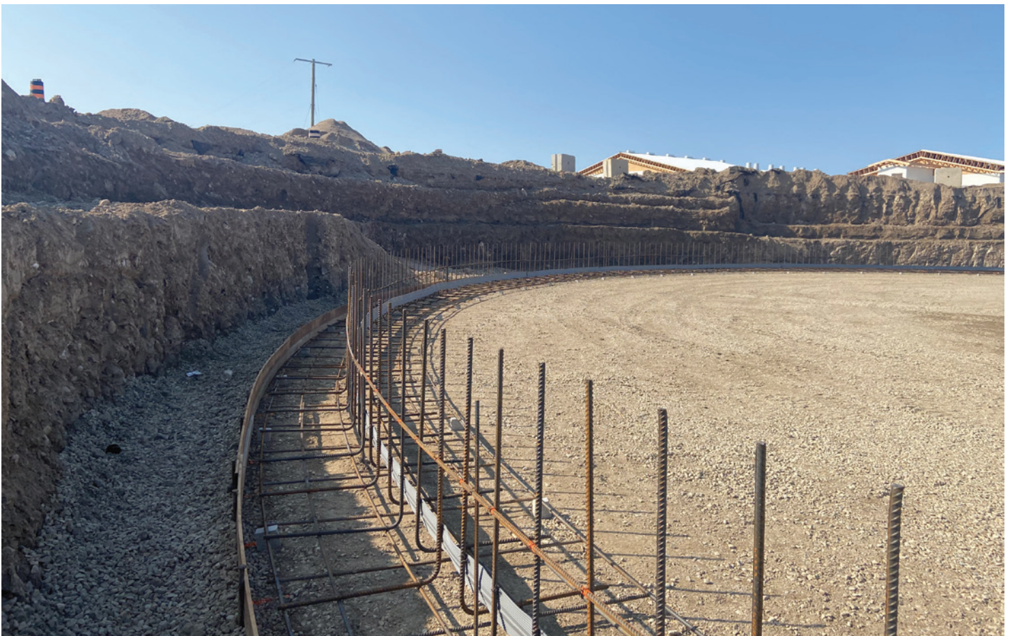
Barres d'armature. © Consultants Lemay & Choinière inc.
