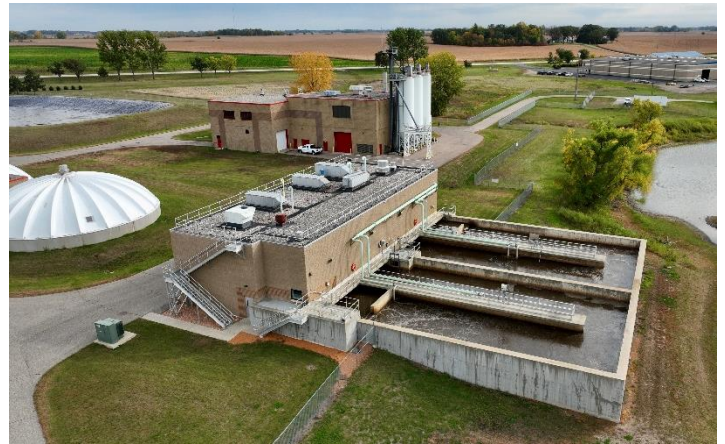
Hutchinson Wastewater Treatment Plant Membrane Bio-Reactor (City of Hutchinson)
