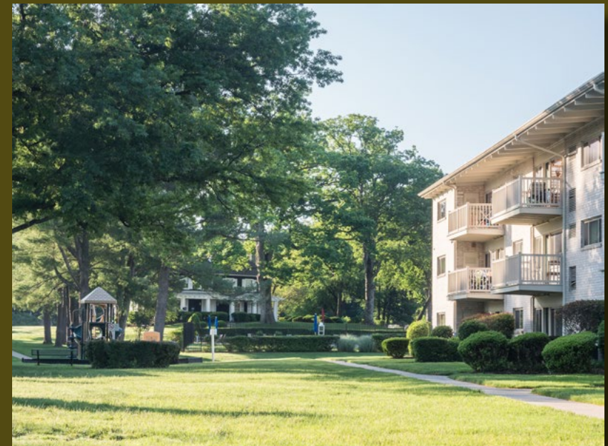
Halpine View Apartments
