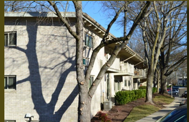
Halpine View Apartments
