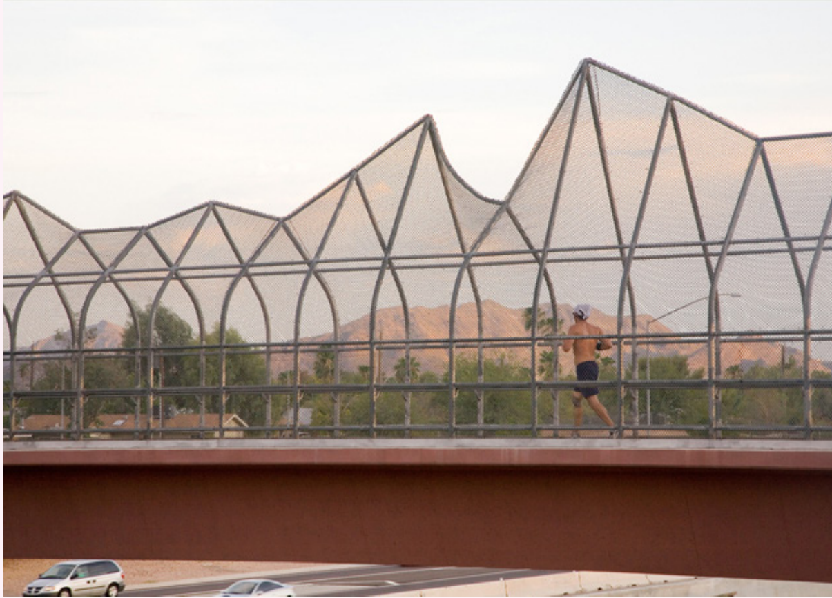
Laurie Lundquist Mountain Pass Pedestrian Bridge 1997
