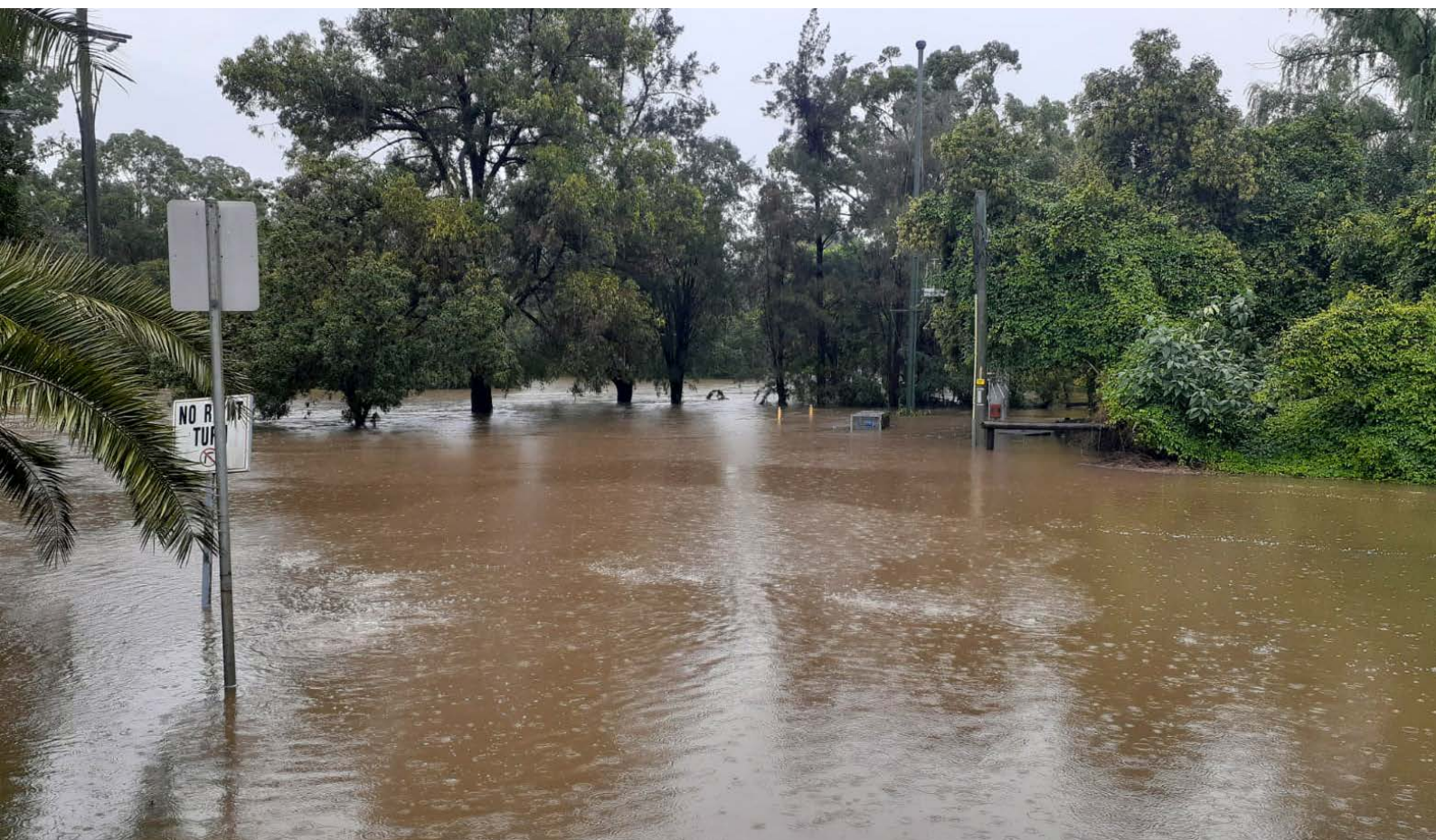
Figure 15: Flooding of the North Richmond Bridge, NSW, 2021.
