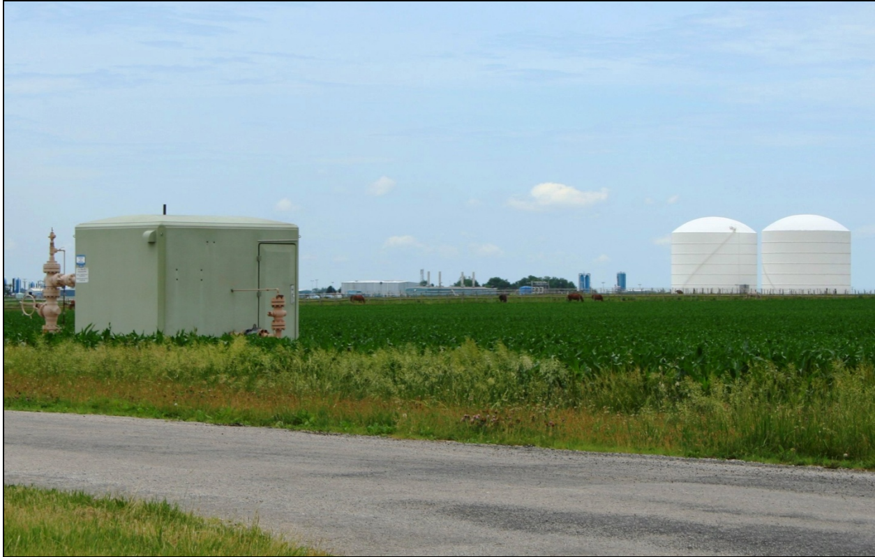
Figure 8 - Fiberglass Housing Surrounding Production Equipment at Gas Storage Field in Midwest United States (Ref. 12) (Photo credit Wikimedia Commons)
