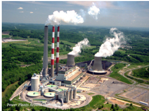
Enclosed coal fired power plant in the northeastern United States (Allegheny Energy) 1
