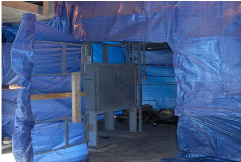
Figure 7: Temporary windbreak created with scaffolding and tarpaulin
