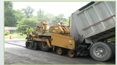
Typical hot mix asphalt paving operation
