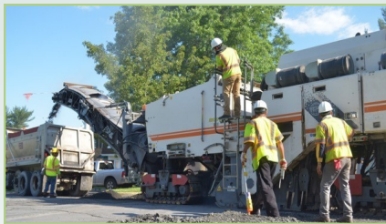
Typical milling operation
