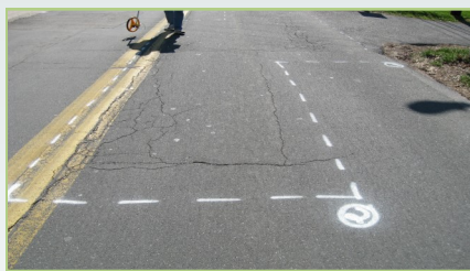
Typical survey paint markings
