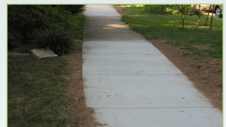
Completed sidewalk repair
