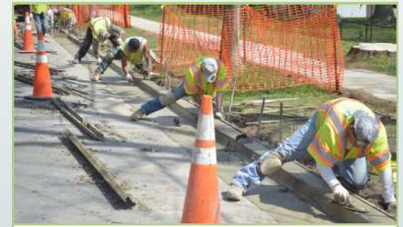
Concrete is smoothed and finished
