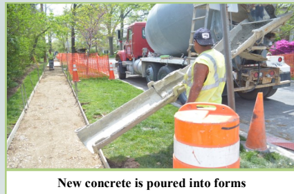
New concrete is poured into forms
