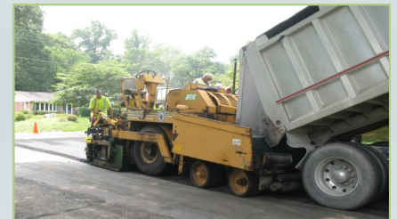
Typical hot mix asphalt paving operation
