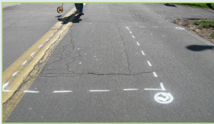
Typical survey paint markings
